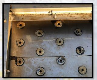
Limescale on cooling tower nozzles
