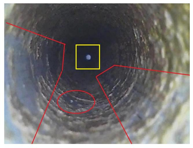
Removing the carbonate layer from the wall of the heat transfer tube using metal brush. Red sectors - zones of removed sediments, yellow sector - clean section at the end of the tube.
