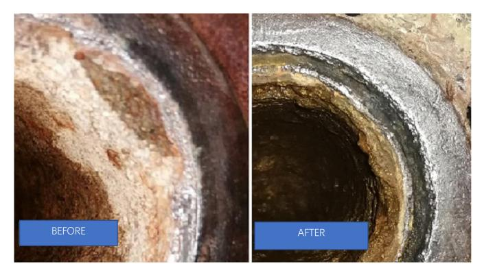
Comparison of the state of the inner surface of the the industrial water supplying pipe at the beginning and at the end of the test installation
